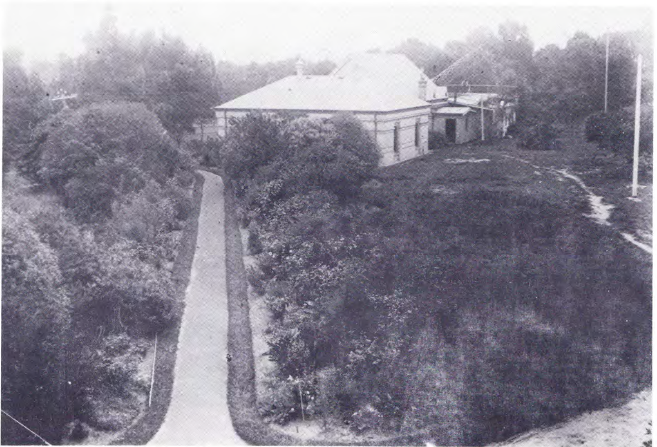
Melbourne Observatory. View of Great Melbourne Telescope Building c.1904-08. The image shows the planting around the Great Melbourne Telescope Building carried out c.1905 following additions to the structure. (Print from glass plate held by Mr Lance Woodhouse, grandson of G. H. Woodhouse, Assistant at the Observatory 1904-44.)
